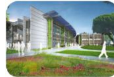
Energy Management for Commercial Buildings
